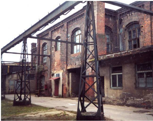
Vankovka factory before.
